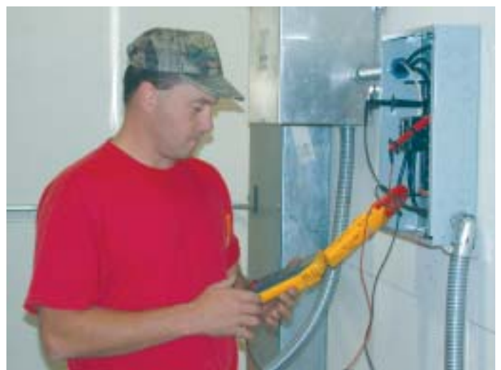
Clark Electric Master Electrician Jim Mertens checks on an electric service for problems.
